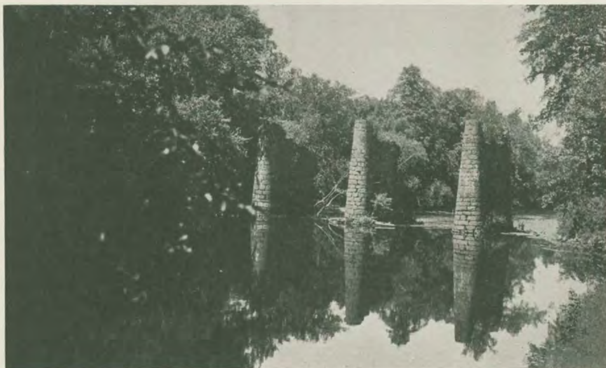
THREE NORTHERLY PIERS OF THE AQUEDUCT OVER FARMINGTON RIVER JUST NORTH OF FARMINGTON ON ROUTE 10. AQUEDUCT HAD 7 SPANS, EACH 40 FEET LONG, 30 FEET ABOVE THE RIVER.
