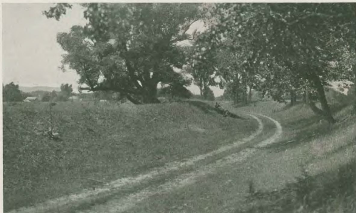
THE GREAT FILL OVER TEN-MILE BROOK AT MILLDALE. HERE IS WHERE A FARMER CUT THE BANK TO FLOOD HIS NEIGHBOR'S LAND. JUST SOUTHWEST OF THE INTERSECTION OF THE CHESHIRE-SOUTHINGTON ROAD WITH THE MERIDEN-WATERBURY HIGHWAY.
