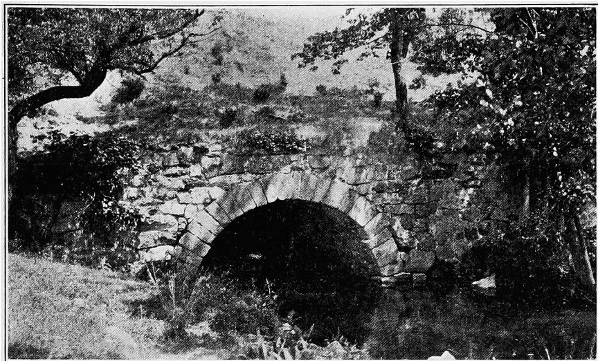
FIG. 5. TYPICAL STONE CULVERT UNDER CANAL.
